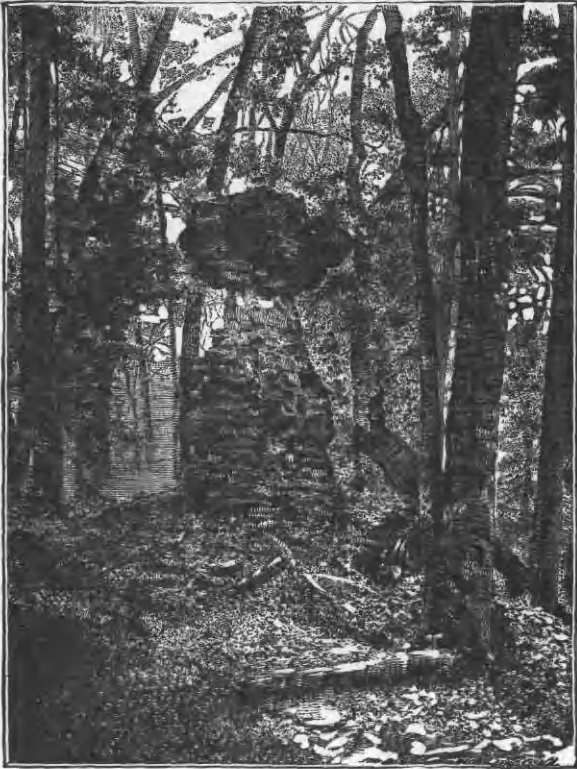
POMPEY'S PILLAR, YELLOW SPRINGS.
