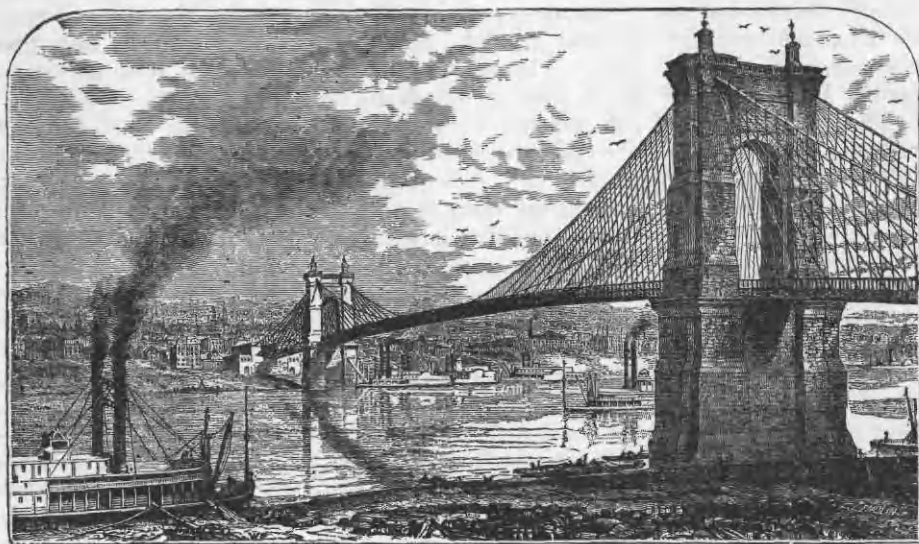
THE SUSPENSION BRIDGE.
